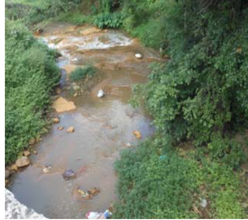
b) Chikhali Nalla at Gangapur Road
